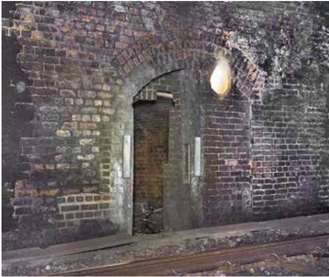
Exterior of a crew room inside the tunnel
